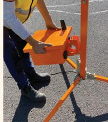
Once the stabilizers are fixed into position, place the Control Box onto the post.
