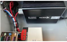
The Battery Charger is located under the shelf in the VMS Control box. The battery charger has an On/Off switch located on the side.
