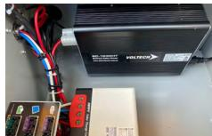
The Battery Charger is located under the shelf in the VSL Control box.
